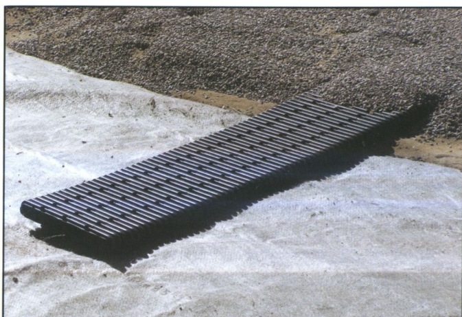
300mm wide Megaflo laid on bidim A5 beneath 6.7mm stone (photo courtesy of Kaytech)
