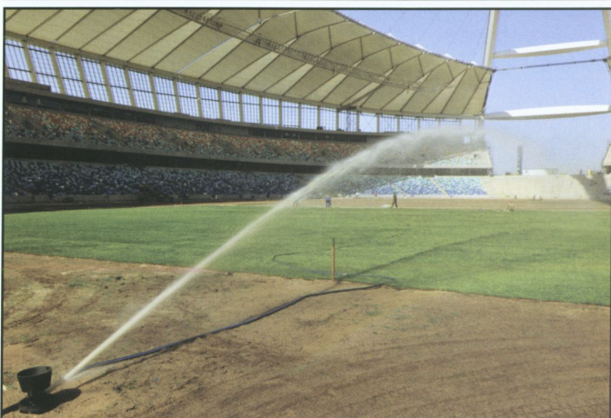
Twelve Perrot sprinklers were installed to irrigate the turf – ten around the perimeter and two in the pitch
