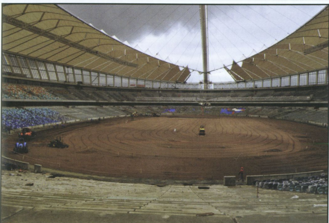
By mid-August 2009 most of the initial growing medium had been laid and the delicate task of shaping the 'turtle back' was underway
