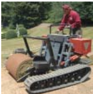
Southern Sod Sales worker uses special "magnum roll" installer
